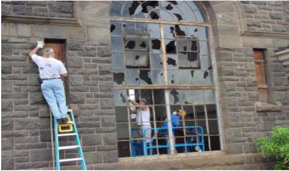
The volunteers painted over graffiti, removed broken window glass, and installed painted boards to cover missing window panes.
