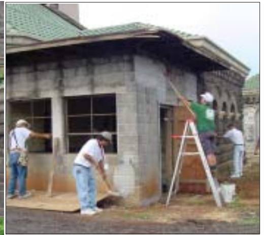
The volunteers painted over graffiti, removed broken window glass, and installed painted boards to cover missing window panes.
